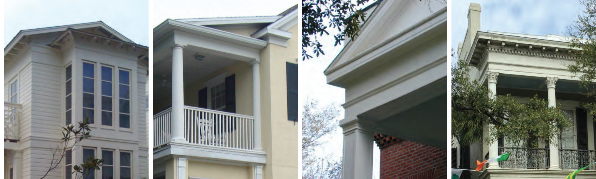
<<<< Cornice enrichments range from the vernacular exposed rafter emulation of mutules and modillions in the far left example to the more refined Greek Revival cornice on the far right. >>>> The most common in Southern Classical are represented by the two examples above - clean closed eave, pediments, and returned eaves at gable ends.
